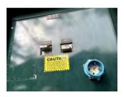
The distribution and control system consist of two motor starters, motor disconnect switches, MultiSmart controls.
