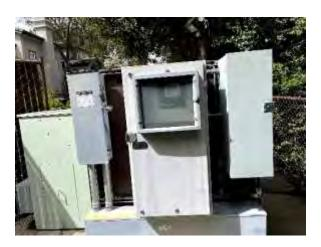
The distribution and control system consists of two motor starters, motor disconnect switches, MultiSmart controls, and hand-off-auto selector switches.
