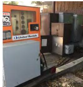
The distribution and control system consist of four motor starters (two not-in-use), motor disconnect switches, MultiSmart controls, and hand-off-auto selector switches.
