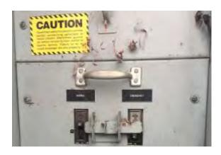
The distribution and control system consist of two motor starters, motor disconnect switches, MultiSmart controls, and hand-off-auto selector switches.
