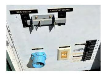
The distribution and control system consist of two motor starters, motor disconnect switches, MultiSmart control, hand-off-auto selector switches.
