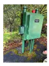
The distribution and control system consists of two motor starters and motor disconnect switches.
