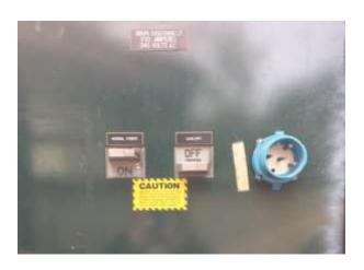
The distribution and control system consist of two motor starters, motor disconnect switches, MultiSmart controls, andnhand-off-auto selector switches.
